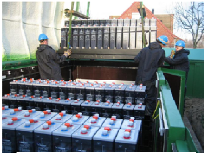
Figure 3: Installation of the Battery Banks
