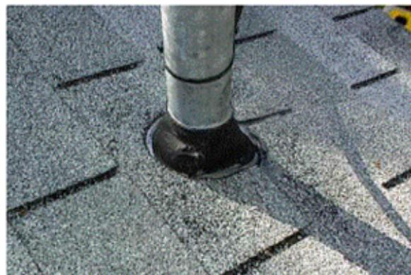
**Figure 6 - Typical installation of rubber roof gland seal.**
