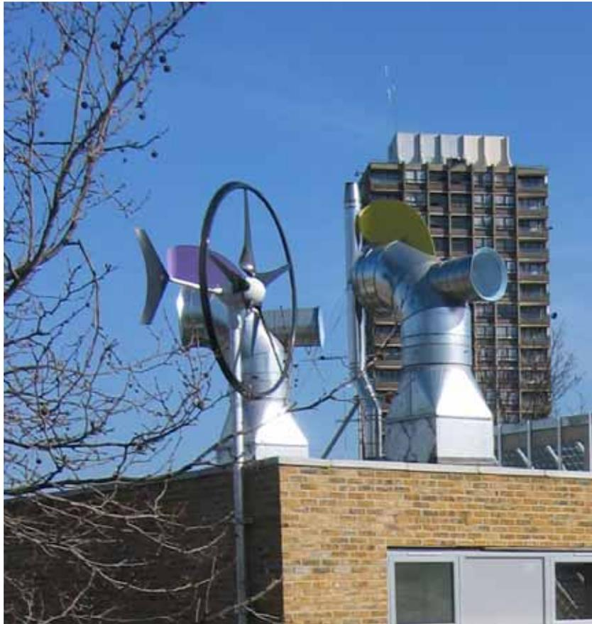
**Figure 1 - Installed Swift Rooftop Wind Energy System**
